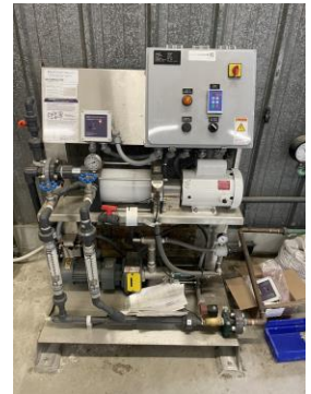
Figure 1: Belt-press, City of Martinez WTP and Polyblend® installed in May 2024
