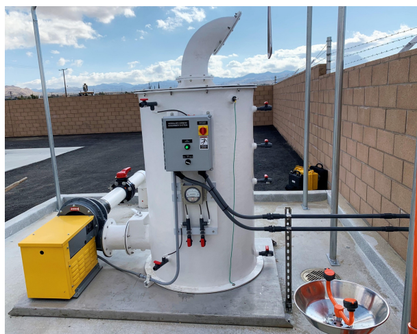
IMS Modular Carbon Odor Control System (MCS-0300) installed at the Paxton Pump Station at the Intersection of Paxton & Balsa Ave
