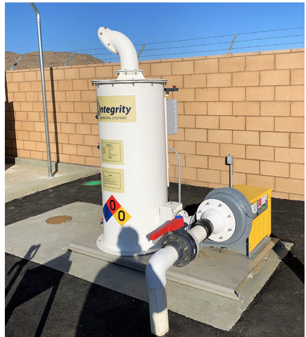
IMS Modular Carbon Odor Control System (MCS-0200) installed at the Barron Pump Station at the Intersection of Barron Ave & Yucca Mesa Rd
