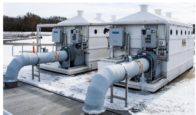
I-BOx® 8015 Biological Odor Control Systems Installed in 2015
